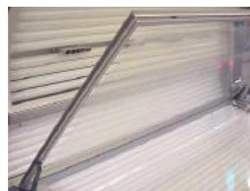
Fig. 3.5 Tilting the base pane
